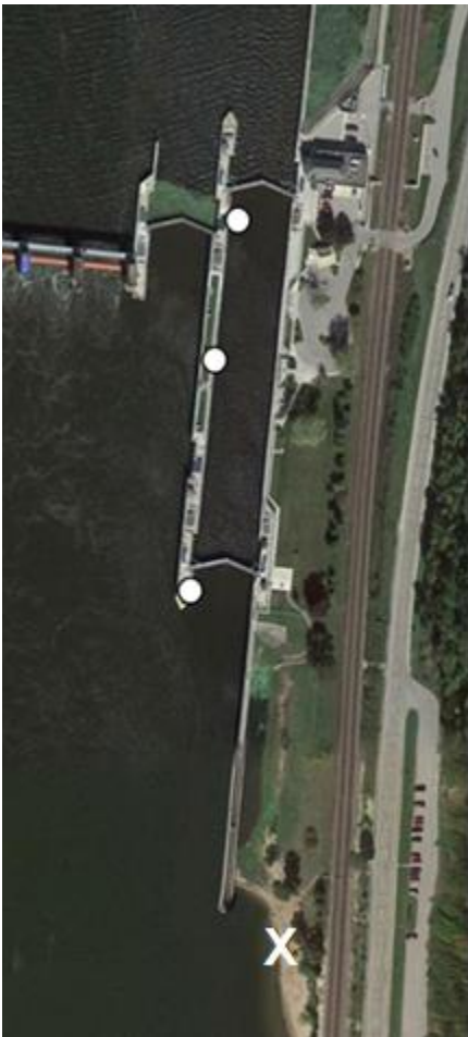
Figure 4: Aerial photograph of the lock at Lock and Dam No. 8 depicting the surgery and release site (white X) and acoustic receivers (white dots).
