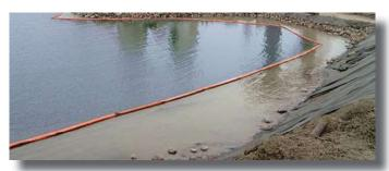
Boat ramp construction requires erosion-control measures, such as a floating silt fence (pictured above) to limit the spread of sediment stirred up by construction. The removal or destruction of aquatic plants to install a boat ramp is an activity regulated by the DNR. If your plans affect aquatic vegetation, please contact a regional DNR Fisheries office because a permit may be required under the Aquatic Plant Management Program.
