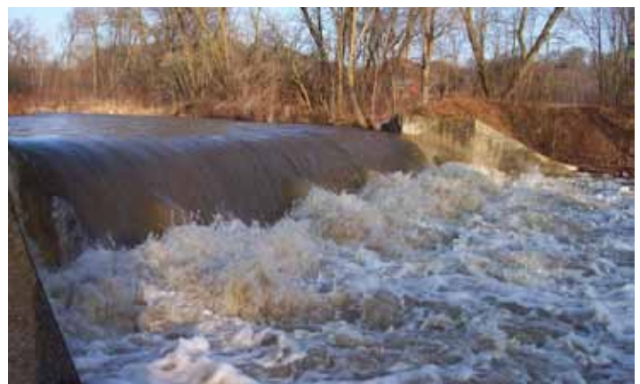
Figure 16. High Island Creek carp dam. Credit DNR EWR.
