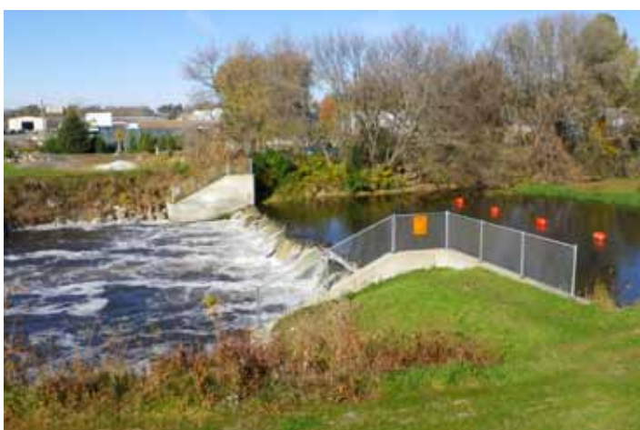
Montevideo Dam on the Chippewa River days before it was modified for fish passage in 2012. Credit DNR SHP.
