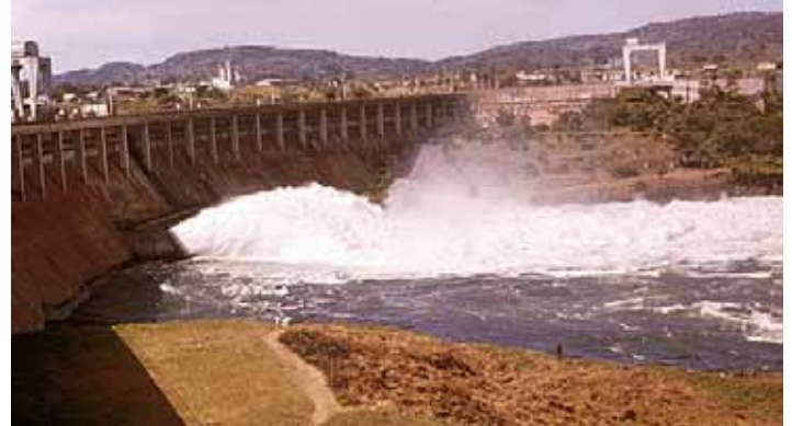
(top) A drawing of Ripon Falls, the natural outlet of Lake Victoria, by explorer John Hanning Speke, courtesy of Princeton University Library. (bottom) Owen Falls Dam/Nalubaale Power Station. Credit USDA Foreign Agricultural Service.
