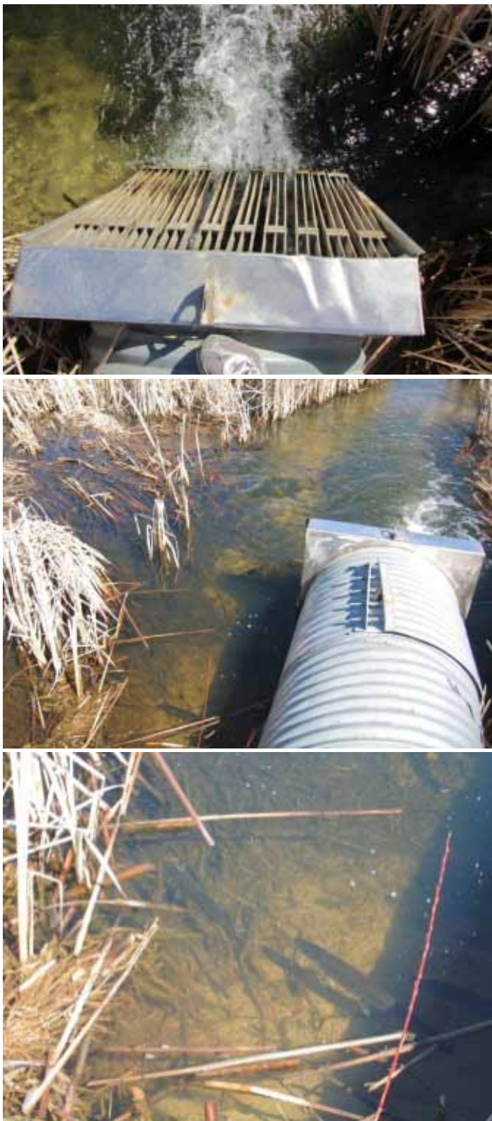
Figure 15. (top & middle) A fairly ubiquitous barrier on smaller streams and lake outlets are carp screens. These physical barriers often create high velocities which further impede fish passage. (bottom) Northern pike blocked by the barrier. Credit DNR SHP.
