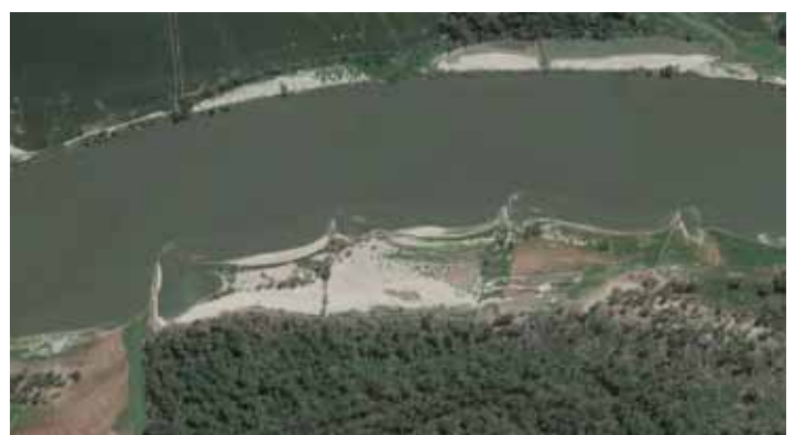
Wing dams that are prevalent in the lower channelized reach in the Missouri River. Google Earth image.
