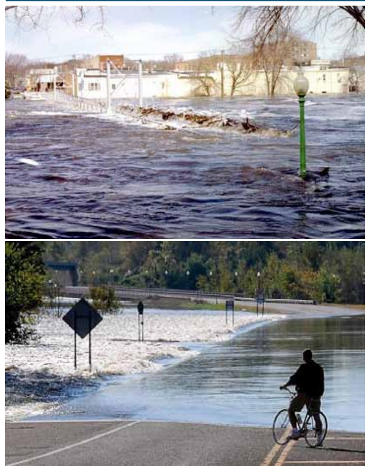
(top) The Minnesota River flooding around an 87-year old pedestrian bridge in Granite Falls. Courtesy of Granite Falls Tribune. (bottom) A bicyclist on Highway 22 south of St. Peter observed the floodwater from the nearby Minnesota River flowing across the roadway. Credit DNR SHP.
